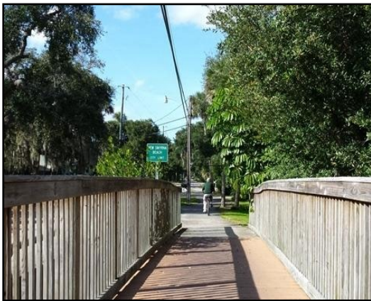
Clay-Duval Trail bridge
