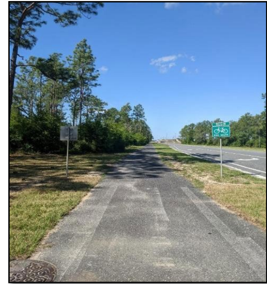
South Street Trail
