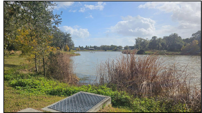
Citrus Hammock Preserve Water Retention Area
