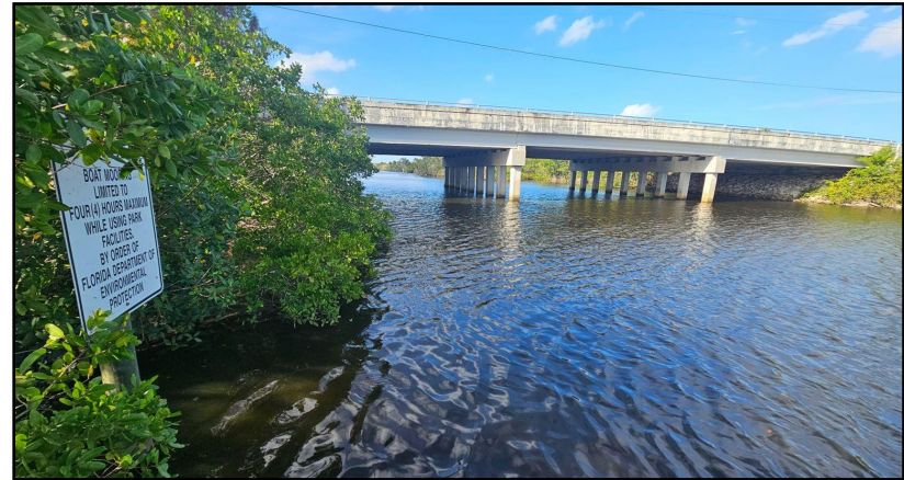
Prima Vista Bridge over St. Lucie River
